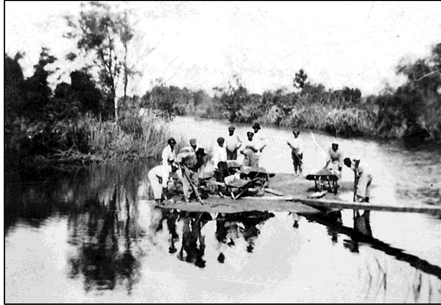
Figure 7.3. Workers repairing a broken rice bank on the Santee Club's Washo Plantation after a hurricane, July 1916. Flood waters had washed much of the bank into the adjacent canal leading from the Santee River, which is in the background of the picture, out of sight. Source: private collection.
